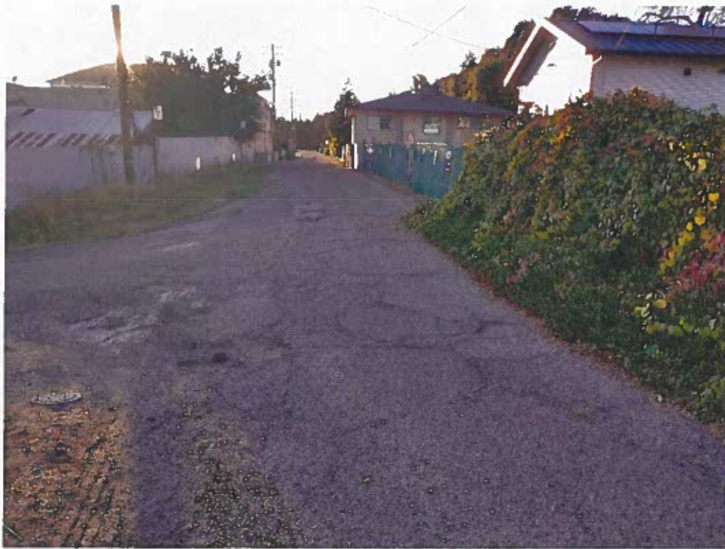
Photo 3 – Looking West on 1st Street from B Street
