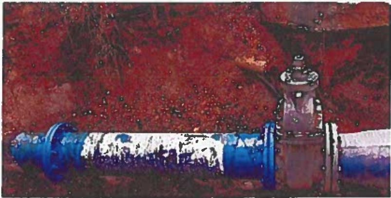
Figure 2-1: Example Infrastructure Repair Work in Isleton
