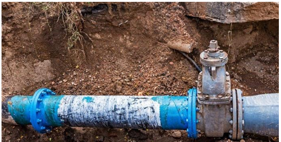
Figure 2-1: Example Infrastructure Repair Work in Isleton
