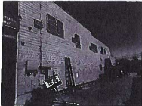
note mounted swamp cooler
