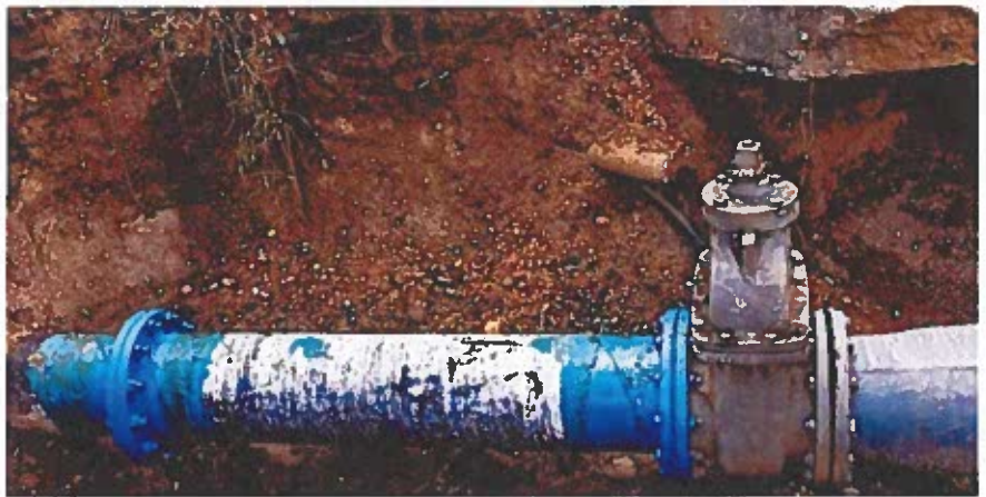
Figure 2-1: Example Infrastructure Repair Work in Isleton
