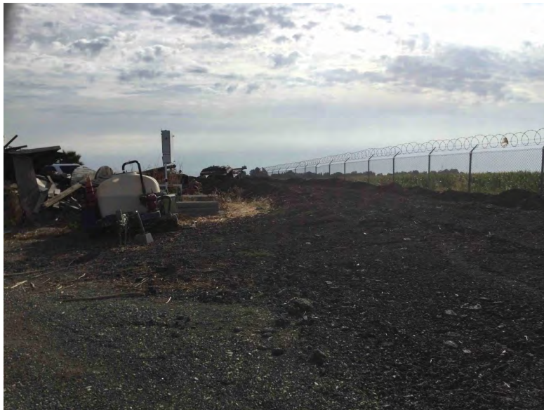
Photo 1. Overview of Corps Yard/Staging Area 1. 8-5-2022
