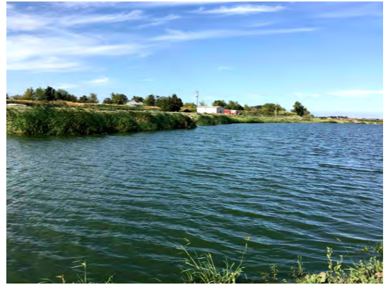
Photo 6. Wastewater treatment pond within WWTP. 8-5-2022
