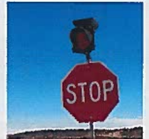
Flashing Beacon at Stop Controlled Intersection
