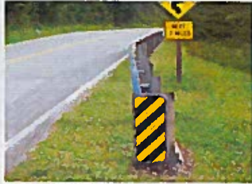
Install Delineators, Reflectors, and Object Markers
