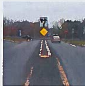
Intersection Splitter Islands (minor road approaches)
