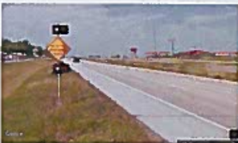
Flashing Beacon as Advanced Warning
