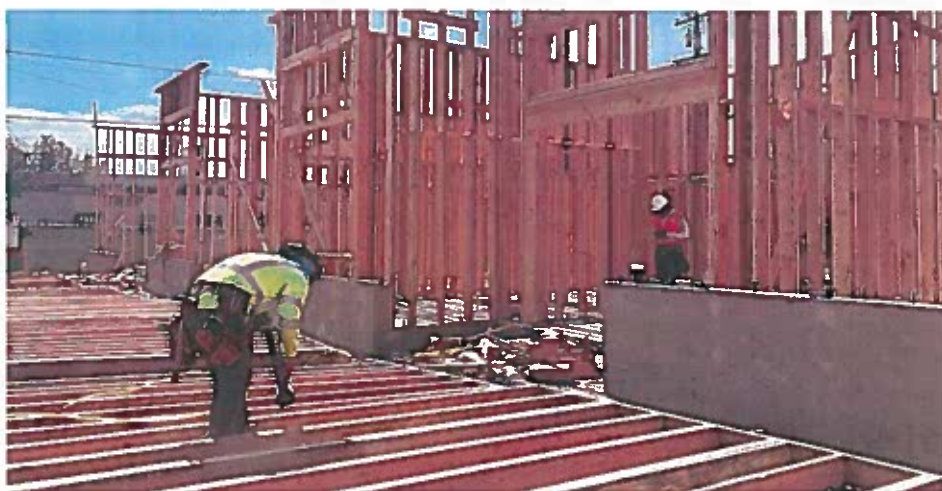
Figure 1-1. Construction of New Housing, photo by Andrew Bowen,
